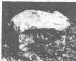
Fig. 254 A 1.3 cu. yd. boulder before mudcapping.
